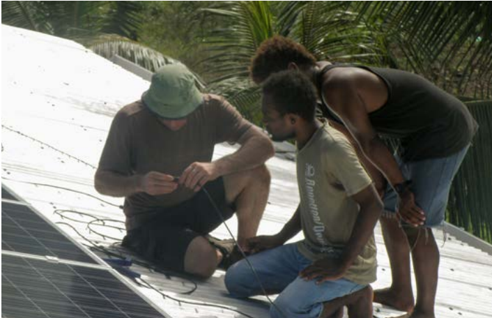
Installing solar power in the Solomon Islands.
