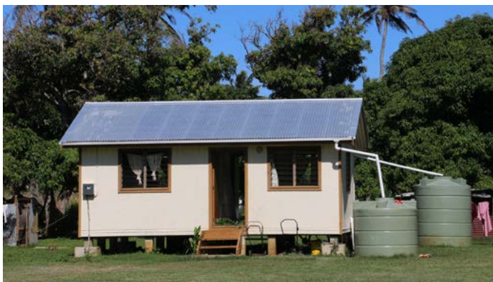
This new house in Ha'apai has been built using cyclone-resistant materials and techniques.
